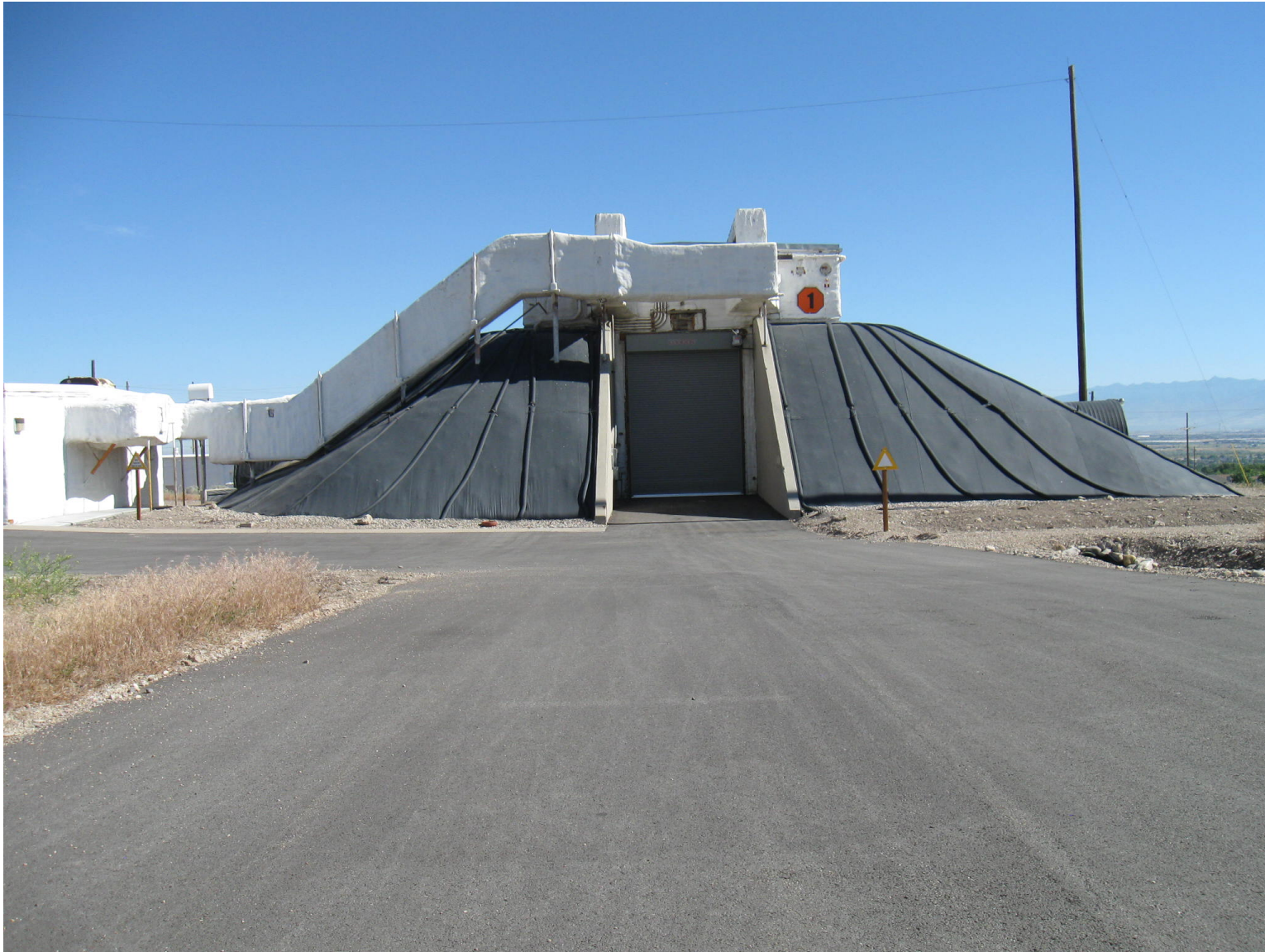
Figure 4-4.8 ES-3 Explosive Storage Building
