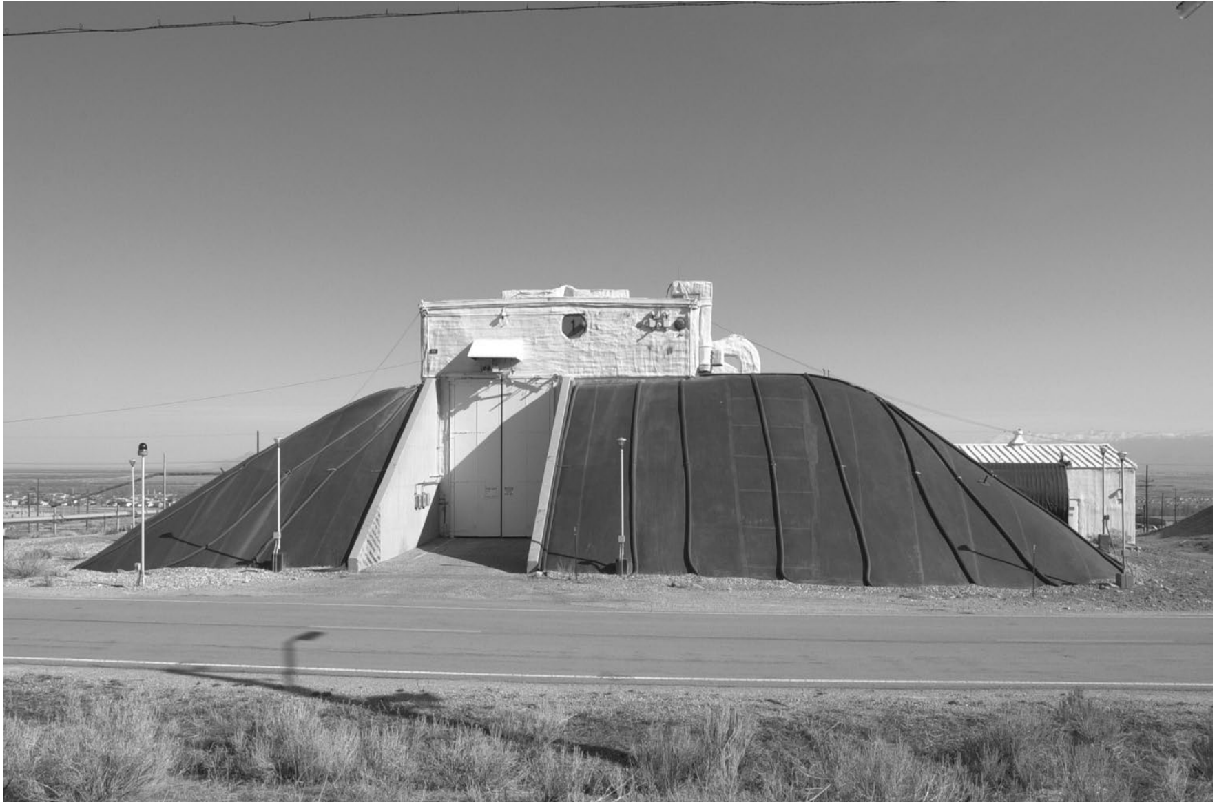
Figure 4-4.5 ES-2 Explosive Storage Building
